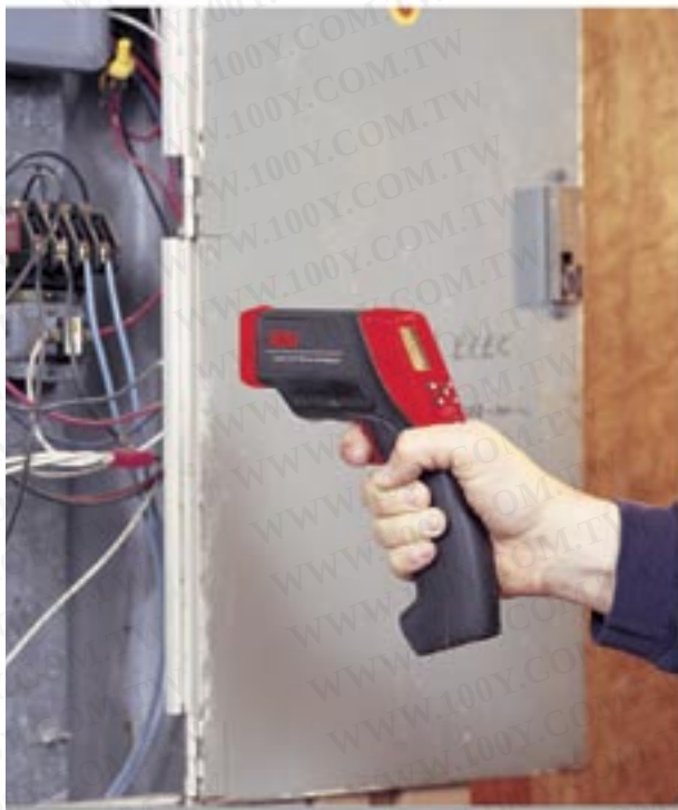
Store temperature measurements for more precise monitoring.
